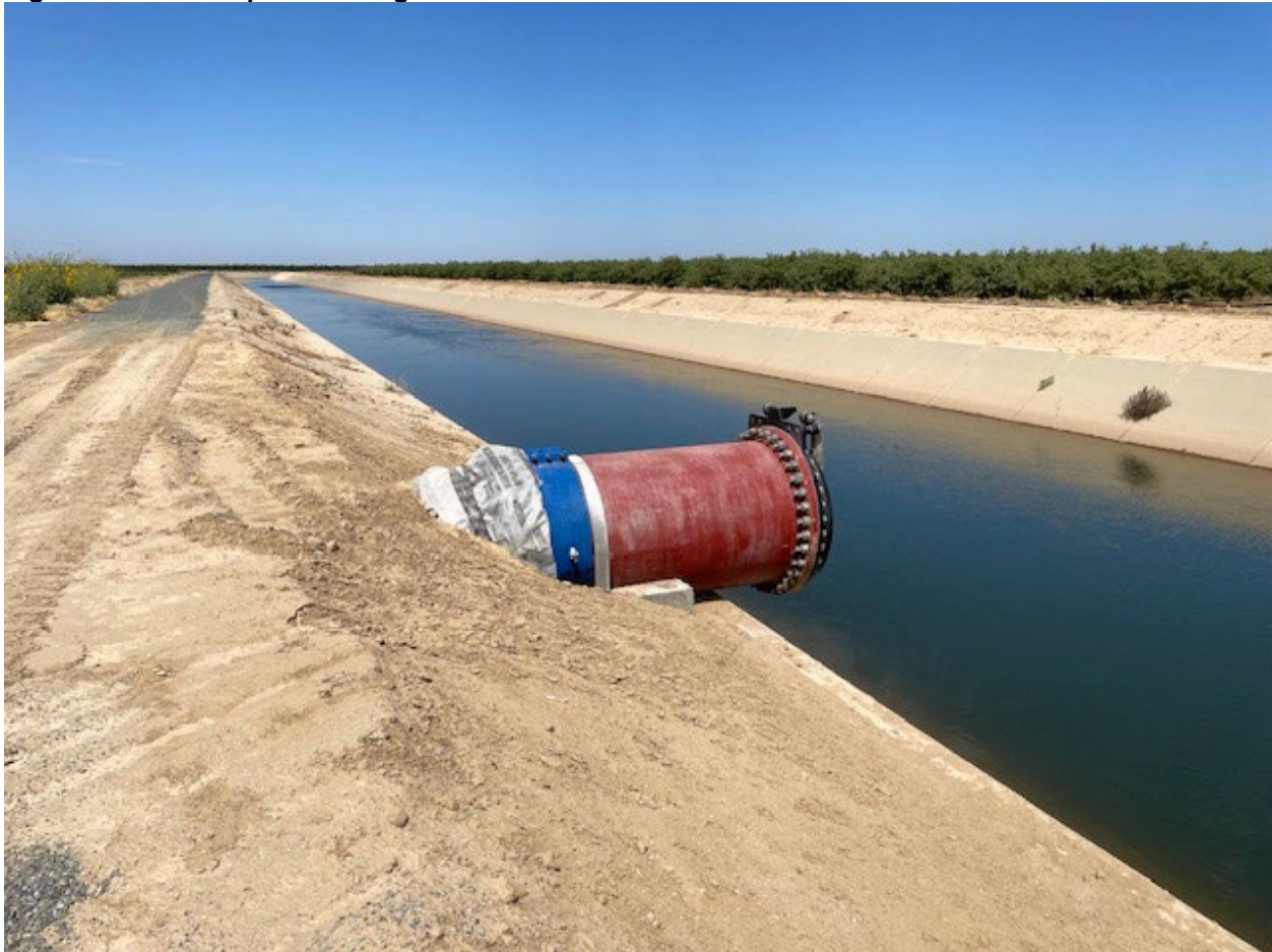
Figure 2-4. Example Discharge Outfall.
