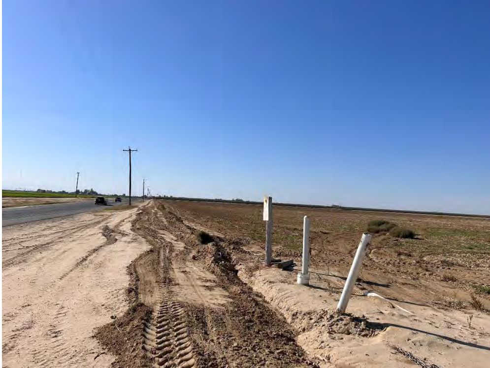
Photo 3. Looking west along Kratzmeyer Road toward the proposed groundwater recharge ponds.
