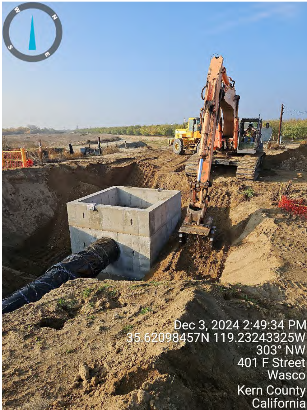
Backfilling concrete vault assembly at 88-29 FKC discharge (12/03/2024)
