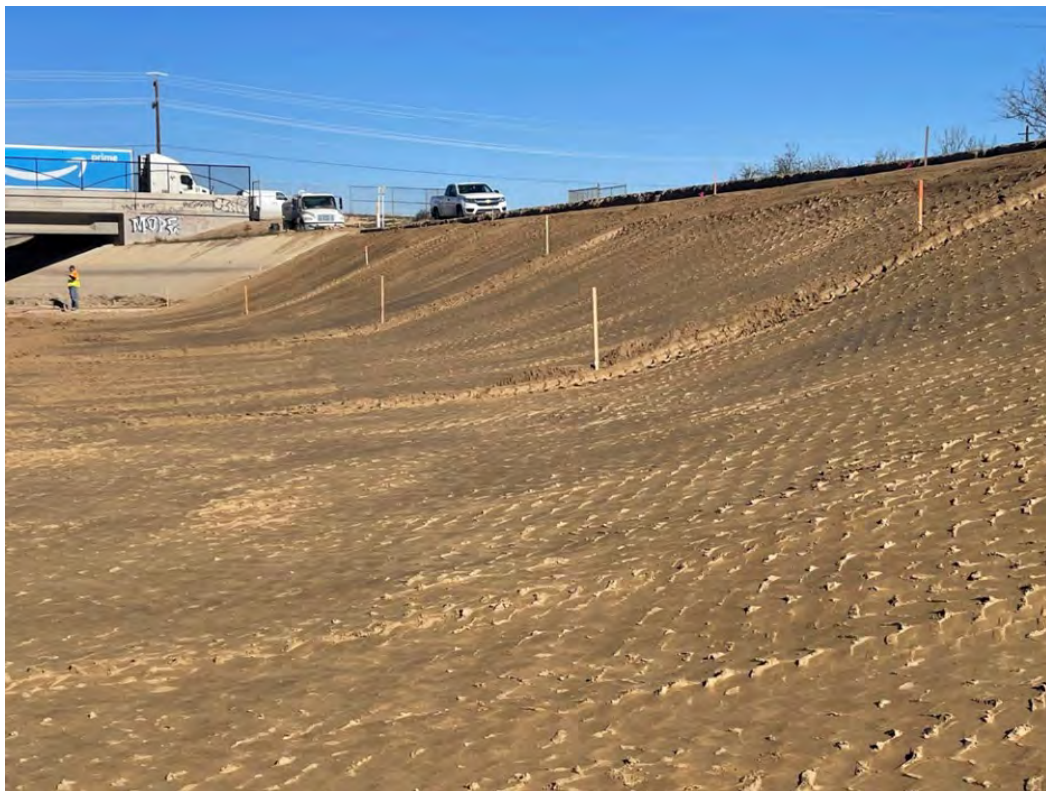
Completed compacted slope prior to finish grading
