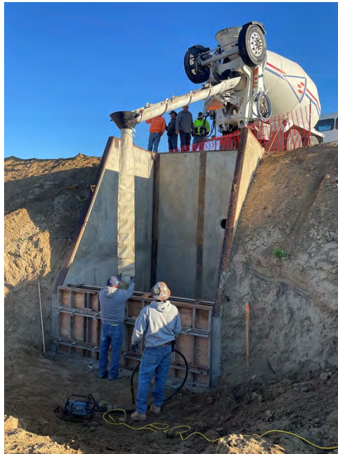
Cut off wall being poured on turnout
