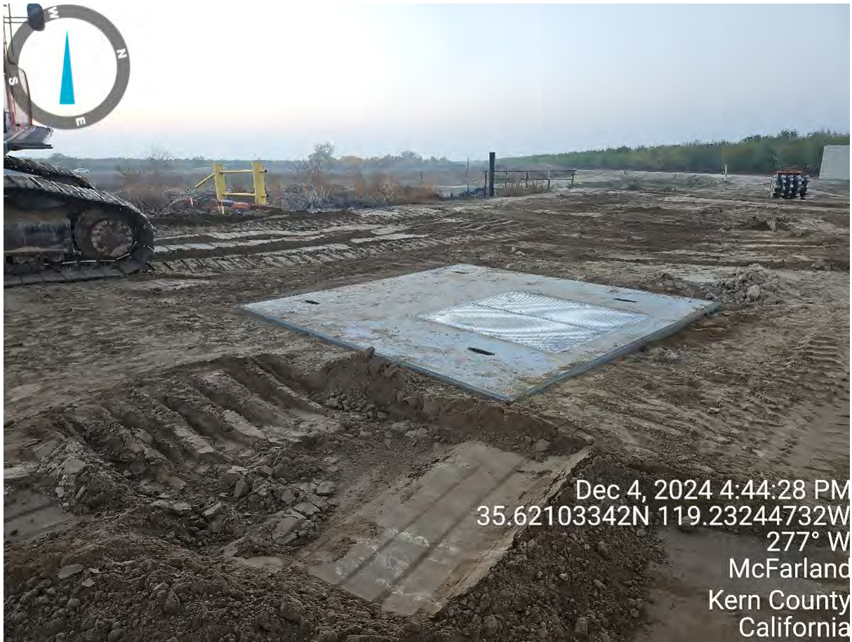
Backfilled concrete vault at 88-29 FKC discharge (12/04/2024)
