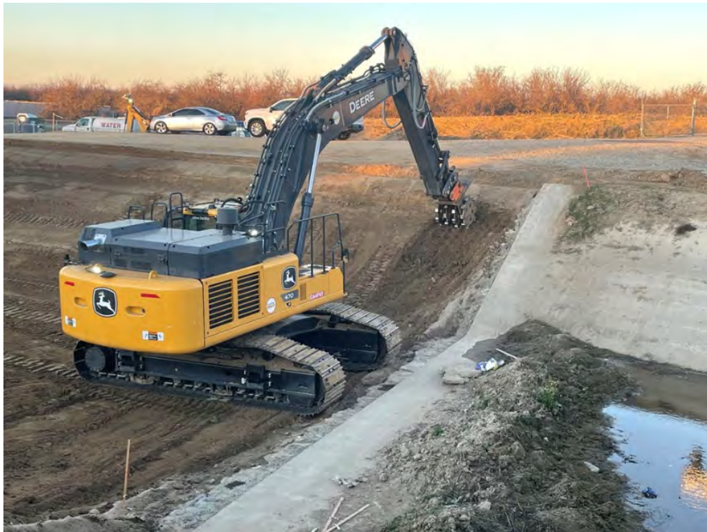
Excavator compacting upper part of side slopes
